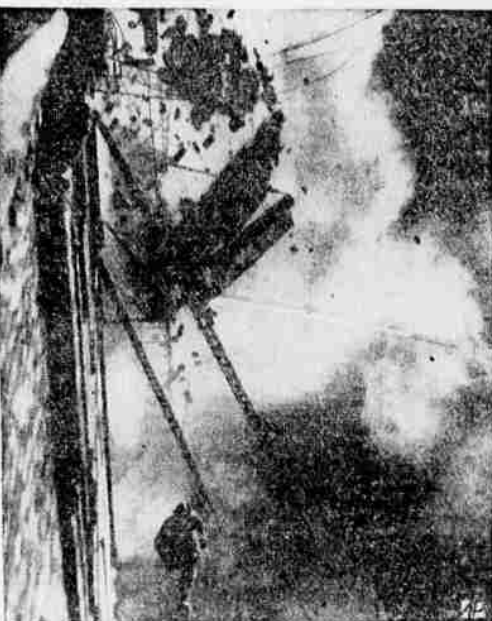
WHEN WALL CRUMBLed —A Philadelphia fireman dashes to safety under crumbling wall which fell on spot where he had stood during October fire at lacquer plant.
