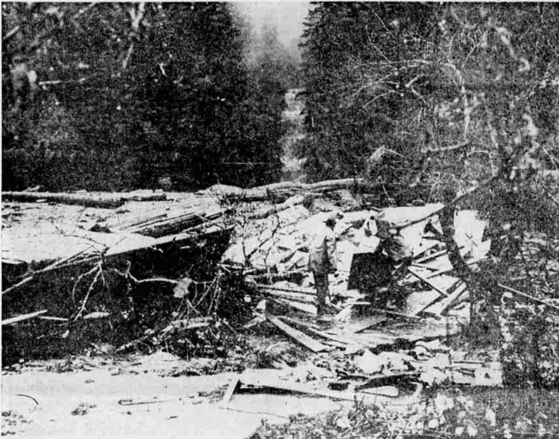
TRAGEDY SCENE —Mud and logs roared down canyon in center background to crush the Neal house, parts of which are scattered in foreground. Waterfall gushes from hillside in canyon where normally there is little water. Camera was pointed uphill from near end of slide. Highway is buried under debris at edge of trees. (Kash photos).
