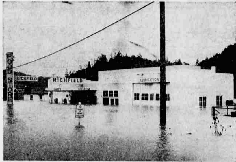
SIX FEET OF WATER was in this grocery store at Myrtle Creek. Barney Root, owner, said most stock was moved high enough to escape damage, but he said he suffered between $1,500 and $2,000 loss. In all, five businesses in this area were under water. Highway 99 is submerged in foreground. (Warren Studio photo).
