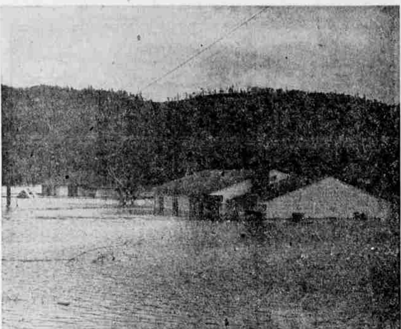
SOME WINSTON HOMES were completely swamped Thursday as the South Umpqua River hit its peak and started to fall. This shot was taken in Winston Section close to river and just north of city. (Paul Jenkins photo).
