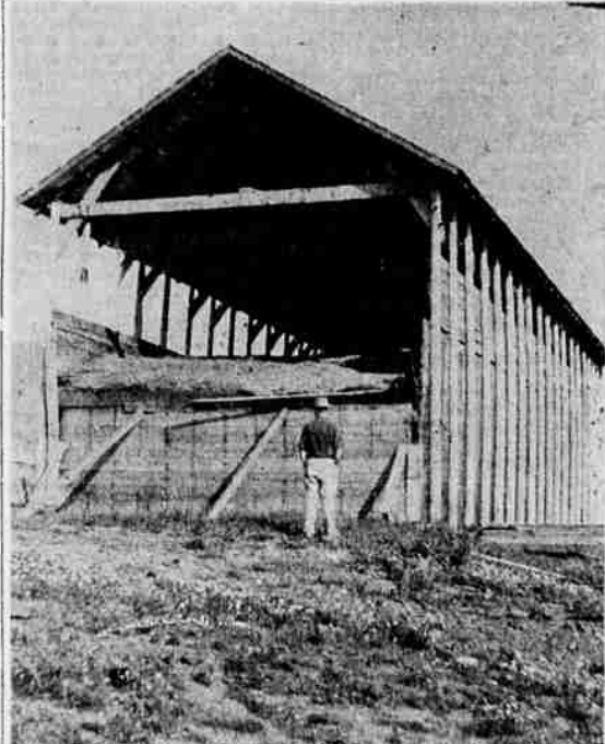
TRENCH SILO —relatively new to Douglas County are trench silos, such as one shown above on the Lawrence Michaels farm, Canyonville. Silo is of pole construction. (Mosher photo)
