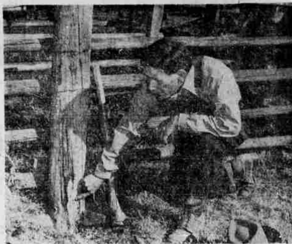
WALT KOCKEN examines a 20-year-old post treated by the salt method.
