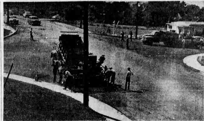
HIGHWAY PAVING CREWS lay down a surface on the new freeway interchange at Harvard Avenue. The new freeway is expected to be opened to traffic before Oct. 1, upon completion of the Shady Bridge south of Roseburg. (Paul Jenkins photo).
