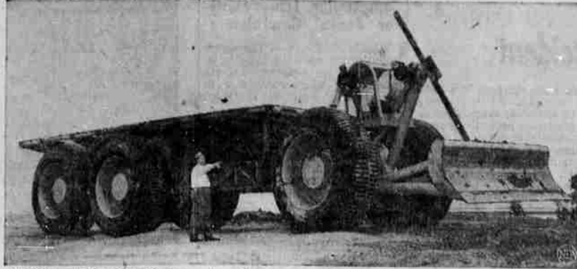
JUNGLE JUGGERNAUT —The automotive monster pictured above is a "Tree Crusher," being tested at Longview, Tex., where it was built by R. G. LeTourneau, Inc. The jungle destroyer travels on the largest rubber tires in the world—10 feet in diameter and 4 feet thick. The 120,000-pound machine is so light on its feet it can roll over a match without breaking it. Yet, in its work of uprooting heavy trees and underbrush, it packs three times the wallop of an M-24 tank. Each of the six wheels has its own electric motor.
