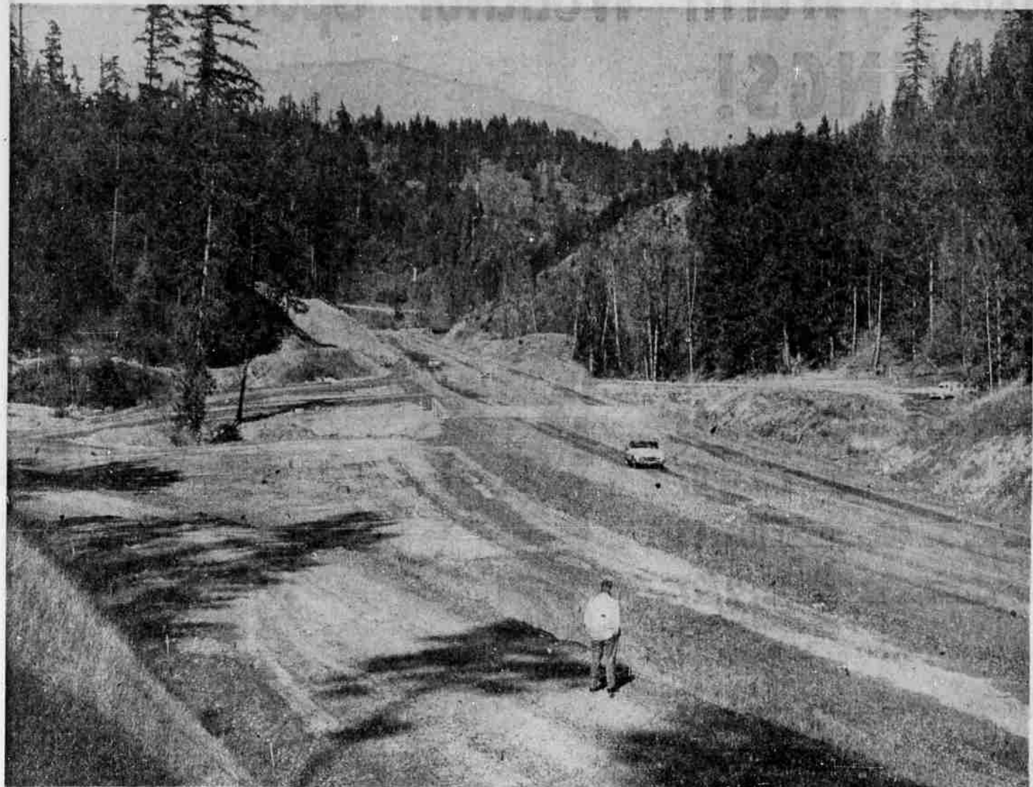
RELOCATED PACIFIC HIGHWAY followed floor of Curtis Creek Canyon through northern part of Anlauf-Rice Hill section. Highway width allows grades. County road crosses under highway here. for climbing lane for slow-moving trucks on
