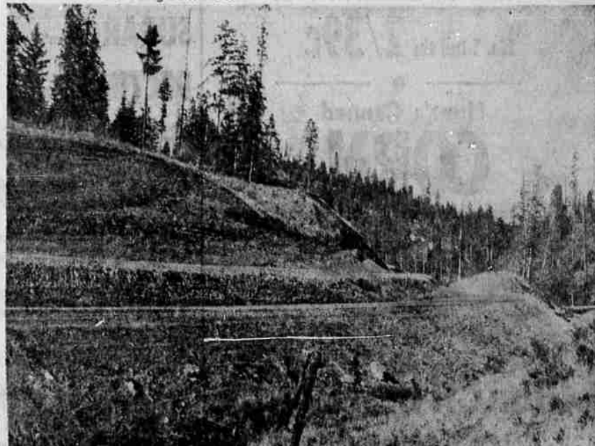
ALLOWANCE FOR FOUR-LANE traffic eventually was made. Shelf above roadway can be cut down with little work to widen roadway.
