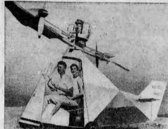
IT FLIES THROUGH THE AIR —This flying scooter will tote 380 pounds through the air for 120 miles, according to the designer. Fueled on premium auto gas mixed with oil, the simple, light helicopter is being made by a Raleigh, N.C. firm, whole or in kits for the do-it-yourselfers. Twin propellers facing in opposite directions spin the 29-foot rotor, which drives the little plane at 60 m.p.h.
