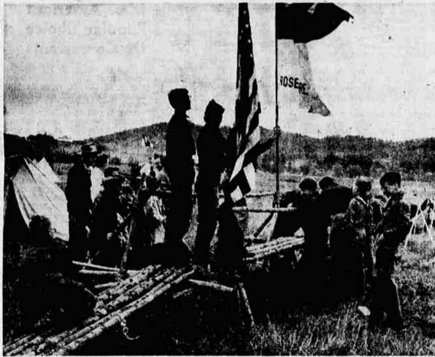
THE ANNUAL CAMPOREE of Douglas Fir District Boy Scouts featured such activities as bench making (top photo), fire building (center) and bridge building (lower). Shown constructing a bench are scouts of Troop 107. Dennis Keebler of Troop 158 is the youngster building a fire despite a drizzling rain. Troop 4 boys are shown proudly planting their flags atop a bridge of poles which they bound together with ropes. (Pictures by Paul Jenkins).
