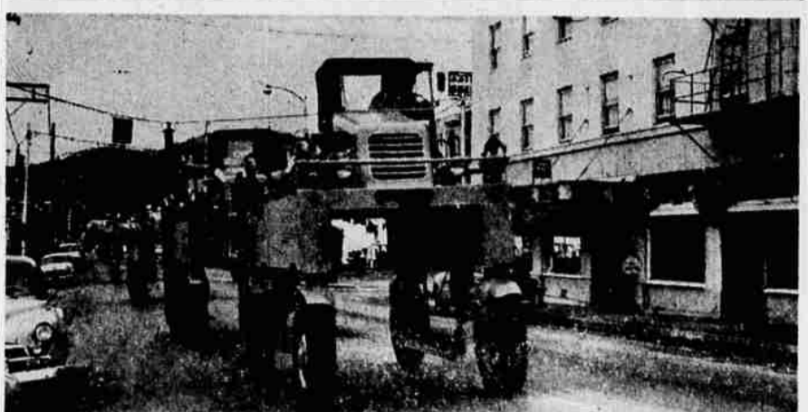
MAKES HISTORY —Rosebush Lumber Co. made history recently by receiving the biggest single delivery of equipment in the history of the Gerlinger Material Carrier Co. plant at Dallas. The delivery included seven material carriers (shown above on the way to the Dillard plant) and three fork lift trucks (not shown). (Photo by Al Monner)
