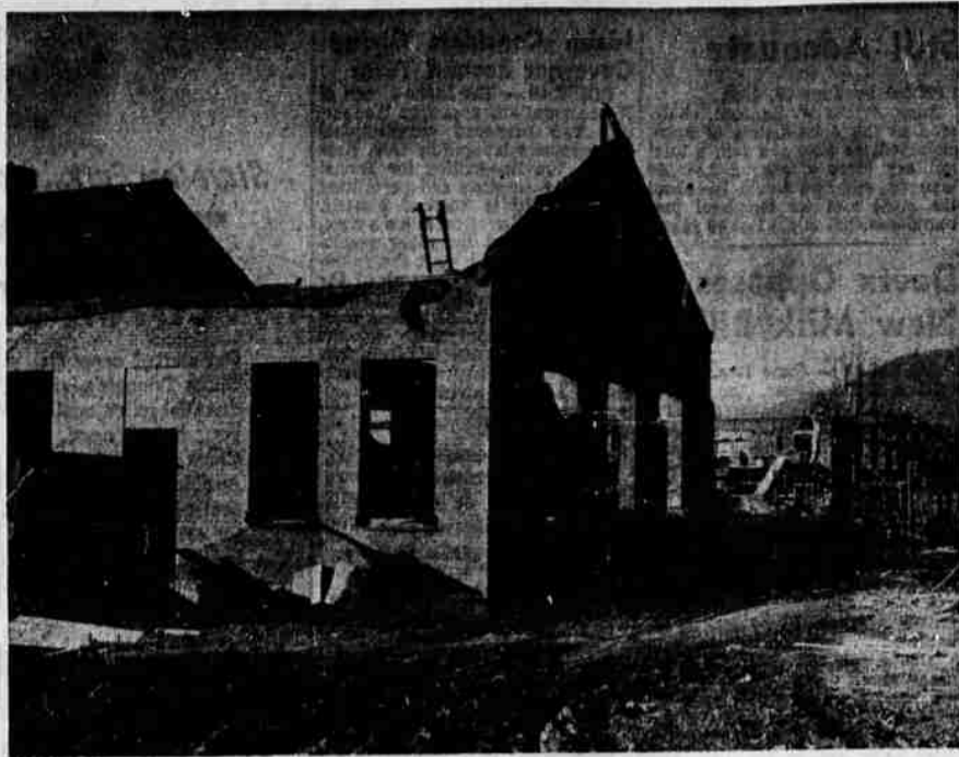
VA EXPANSION GOING UP—Construction is under way on addition to the physical medicine rehabilitation service at the Veterans Administration Hospital in Roseburg. The $125,000 project started in September and will be completed by June. It will add about one-third more space to present buildings occupied by manual arts and occupations therapy sections and will practically double number of patients who will be able to take advantage of this type of treatment. Todd Building Co. is contractor, and supervision is under C. H. Ruehmann, Washington, D. C., VA construction superintendent. (VA photo).
