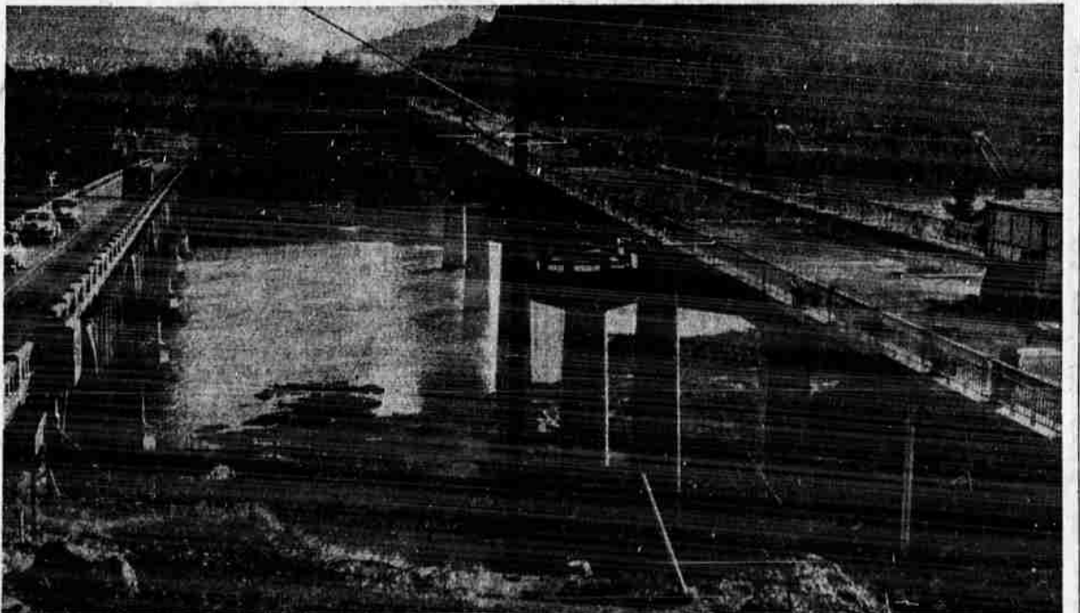
NEW BRIDGE SHAPES UP—Deck on the new Winchester Bridge has been completed, and bridge construction crews are mopping up ends of their work in preparation for completion of the bridge about March 1. The bridge may be put to use about that date, State Highway Engineer R. H. Baldock reportedly is studying feasibility of allowing traffic on relocated highway as far as Garden Valley Road. Meanwhile, the picturesque old bridge at left remains in use for Highway 99 traffic. Deck of new bridge is 30 feet wide and will eliminate cramped space of old bridge. (Paul Jenkins photo)
