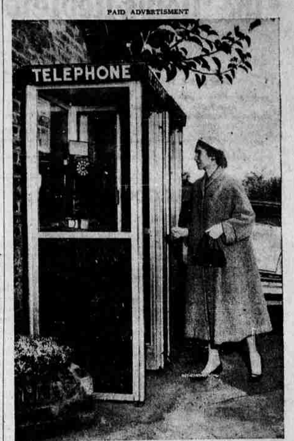
Outdoor telephone booths get new look. Instead of wood, these new models have silvery-white aluminum frames, with big glass panels. They're larger, have better lighting and ventilation. These booths are more convenient to use... cost less to take care of... last longer. They help us bring you more and better telephone service. Pacific Telephone works to make your telephone a bigger value every day.
