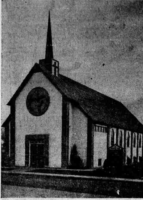
DEDICATION CEREMONIES for the new Apostolic Faith Church will take place Sunday at 3 p.m. when members gather at the newly completed building. Members of Portland congregation and the Rev. Robert Crawford, general overseer, will be present for services. (Photo By Photo Lab.)
