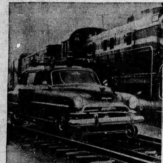
DOUBLE DUTY—This "convertible" automobile owned by Alfred Perlman, president of the New York Central, takes to the railroad tracks near Weehauken, N. J. The car is equipped to ride on rails as well as roads so that Perlman's inspection trips are made easier. The car rides the tracks on oversized pneumatic tires, and has miniature flanged railroad wheels in front and back to keep the car on the tracks. Its speed on the rails is supposedly 35 mph.
