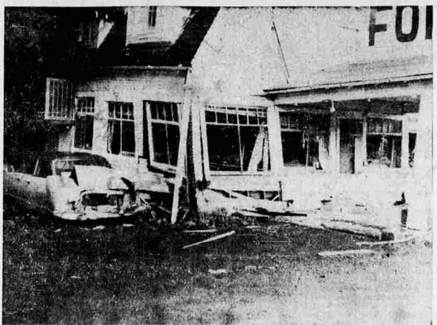
A WELL-KNOWN DOUGLAS COUNTY EATERY was knocked down from its foundations at 5 a.m. Sunday. Complete disorder greeted the owner of Ford's when he came to view the accident caused by a Beaverton motorist. (Ruth Evans photo)
