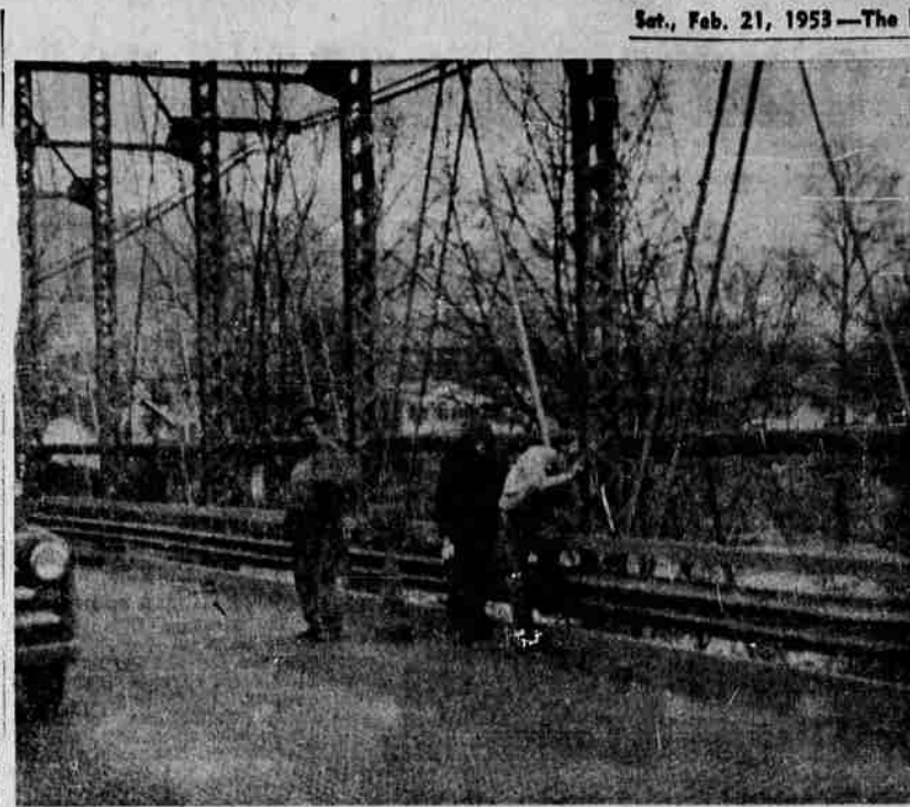
BRIDGEWORK — Douglas County crews meet the challenge of progress with the installation of modern metal sheeting on the Oak St. Bridge to replace the hogwire which was formerly used for protective purposes. (Picture by Paul Jenkins.)
