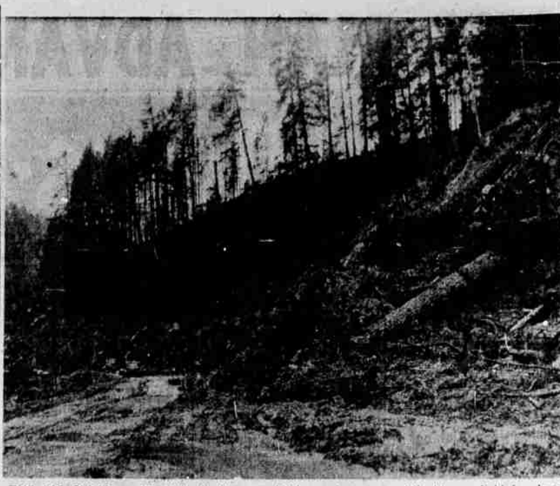
THE BIG SLIDE — The North Umpqua Highway between Idleyld and Mc's place was chewed to pieces by this slide recently which carried trees and gigantic boulders in its wake. The slide closed the highway for a week before this tiny one-way channel was cut through. The present rutted, single-lane passage leaves room for barely one car to pass through at a time. (Staff picture)
