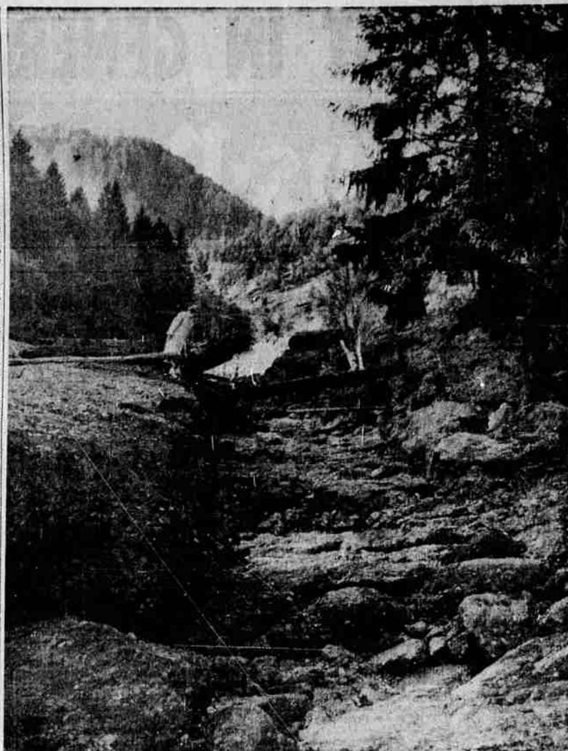
RAMPAGING STREAMS WRECKED numerous roads throughout the County over the weekend. Here's a shot of what used to be the Cow Creek Canyon Road. What looks now like an ordinary rough, rocky stream bed was just a few days back a good gravelled road. Several families live above this section of the road and are forced to walk in and out to Riddle. One man said his car had been trapped on the upper side of the water damage and now a trip into Riddle is a nine-mile hike for him. (Picture by Paul Jenkins)
