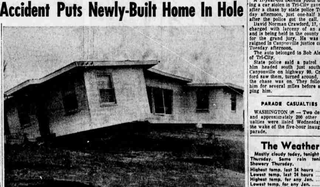
FLOOD DAMAGES HOME —When Al Sanders of Riversdale got up Sunday morning he heard cracking noises. It wasn't long before his new home, which he began last April, looked like this. The rampaging Umpqua River undercut it and the structure toppled over into a six-foot-deep hole. (Picture by Paul Jenkins)
