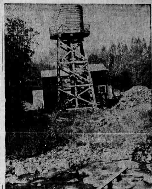
HEADWORKS of new Sutherlin water system is eight miles east of Sutherlin on Calapooia Creek. Unit includes filtering system and chlorinator. Tower provides wash water for filter system.
