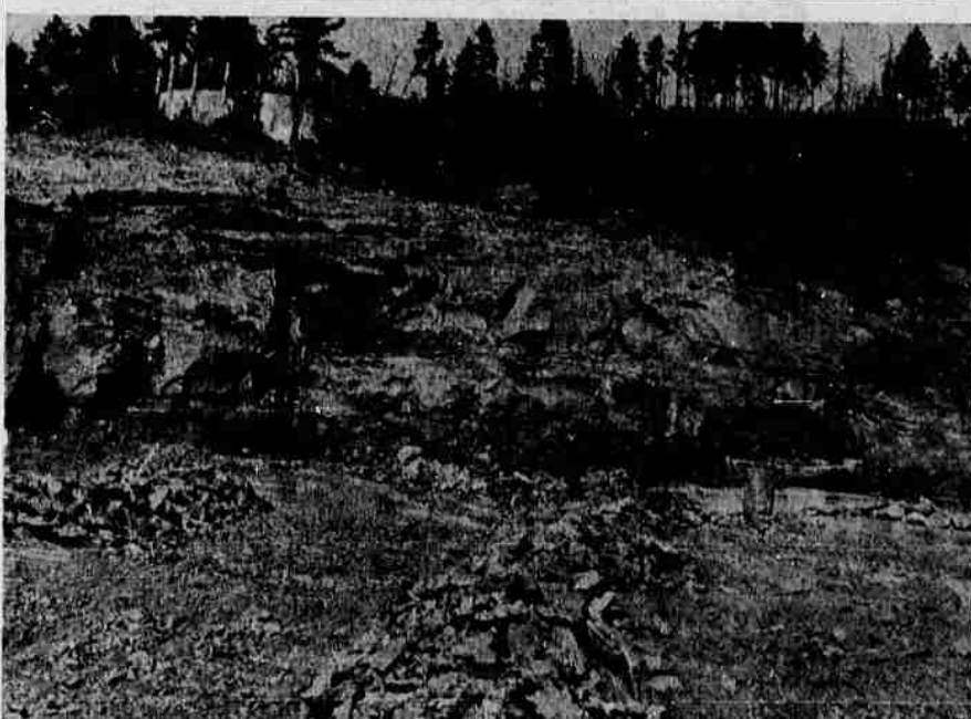
NEW RESERVOIR —Workmen gouge out area atop hill north of Sutherlin for construction of a new 1,125,000-gallon capacity reservoir to serve the city. At top left is ancient 60,000-gallon reservoir built sometime between 1911 and 1925 and still in use. Old 400,000-gallon reservoir was torn out to make way for the new structure.
