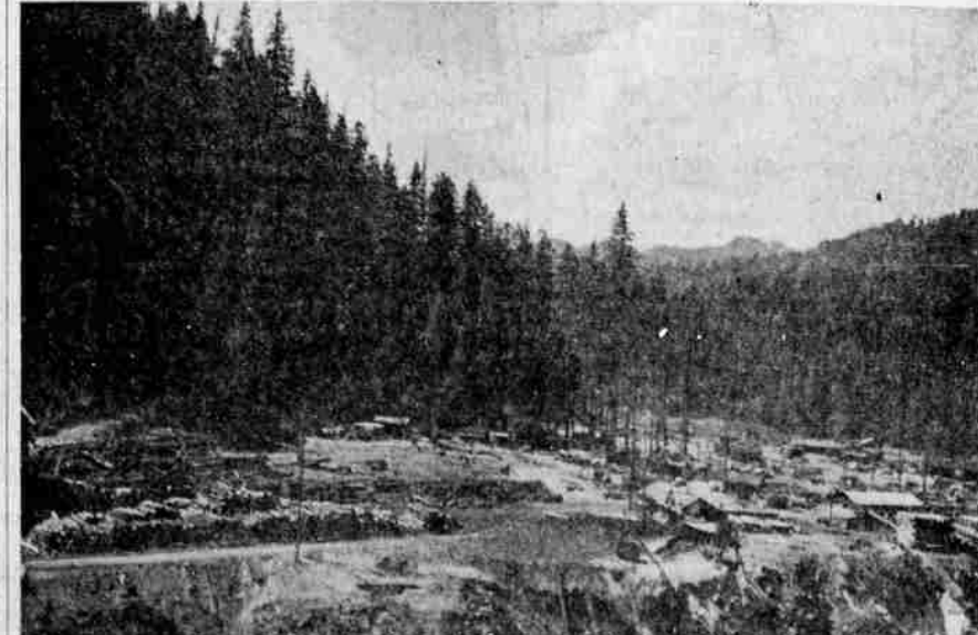
SAWMILL —This sawmill is capable of cutting a million board feet a month. The trees cut on the job are cut into rough lumber to be used for various construction purposes in the development area. The other buildings in the area are the remains of the Soda Springs Construction camp.
