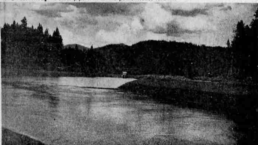
FISH CREEK FOREBAY has a capacity of 60 acre feet and enables water to be ponded for peaking purposes.
