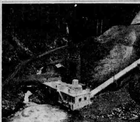
SLIDE CREEK PLANT —This 18,000 kilowatt plant is supervisory controlled (remotely) from the Toketee power house and therefore does not require operating personnel. The water to operate this plant is diverted from the North Umpqua River by a 35-foot high diversion dam and is carried to the turbine through a series of timber flumes and concrete lined canals, which ultimately turn the water into a 12-foot diameter steel penstock, which directly joins the power plant.
