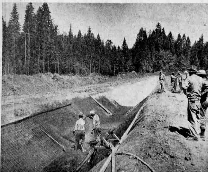
FISH CREEK CANAL —This is a section of the concrete-lined canal that carries water to the Fish Creek power plant. There is 15,681 feet of canal, plus 7,778 feet of timber flume. The workmen are applying concrete under pressure over the steel reinforcing mats. Water carried by this canal empties into the forebay shown above.
