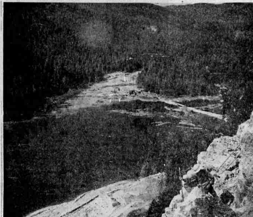
CLEARWATER NO. 2 PLANT SITE is seen from a vantage point 750 feet above the Toketee pond. The open ground across the water is a gravel pit which supplies much of the aggregate for construction purposes. Workman in foreground is knocking loose rock down in preparation of the steel penstock footings on this perpendicular cliff.
