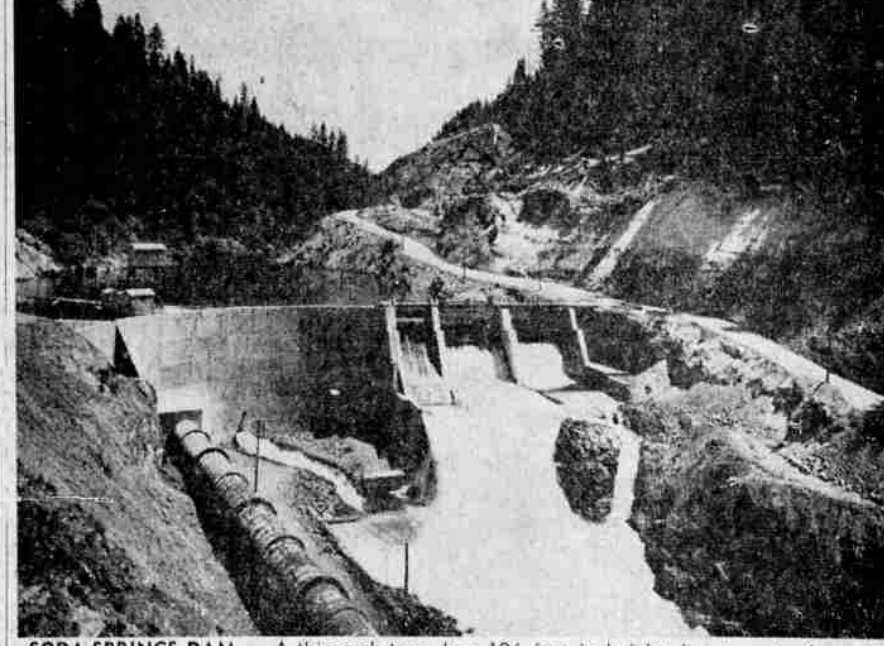
SODA SPRINGS DAM —A thin arch-type dam 126 feet in height diverts water from the North Umpqua River and sends it through 2,085 feet of steel pipe 12 feet in diameter to the power house turbine.
