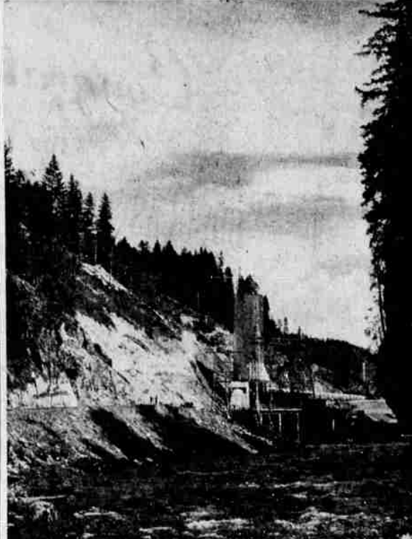
SODA SPRINGS POWER PLANT —The third plant completed in the Umpqua development is the 11,000 kilowatt Soda Springs plant. This is an out-door-type plant and is also supervisory controlled from the Toketee power house.
