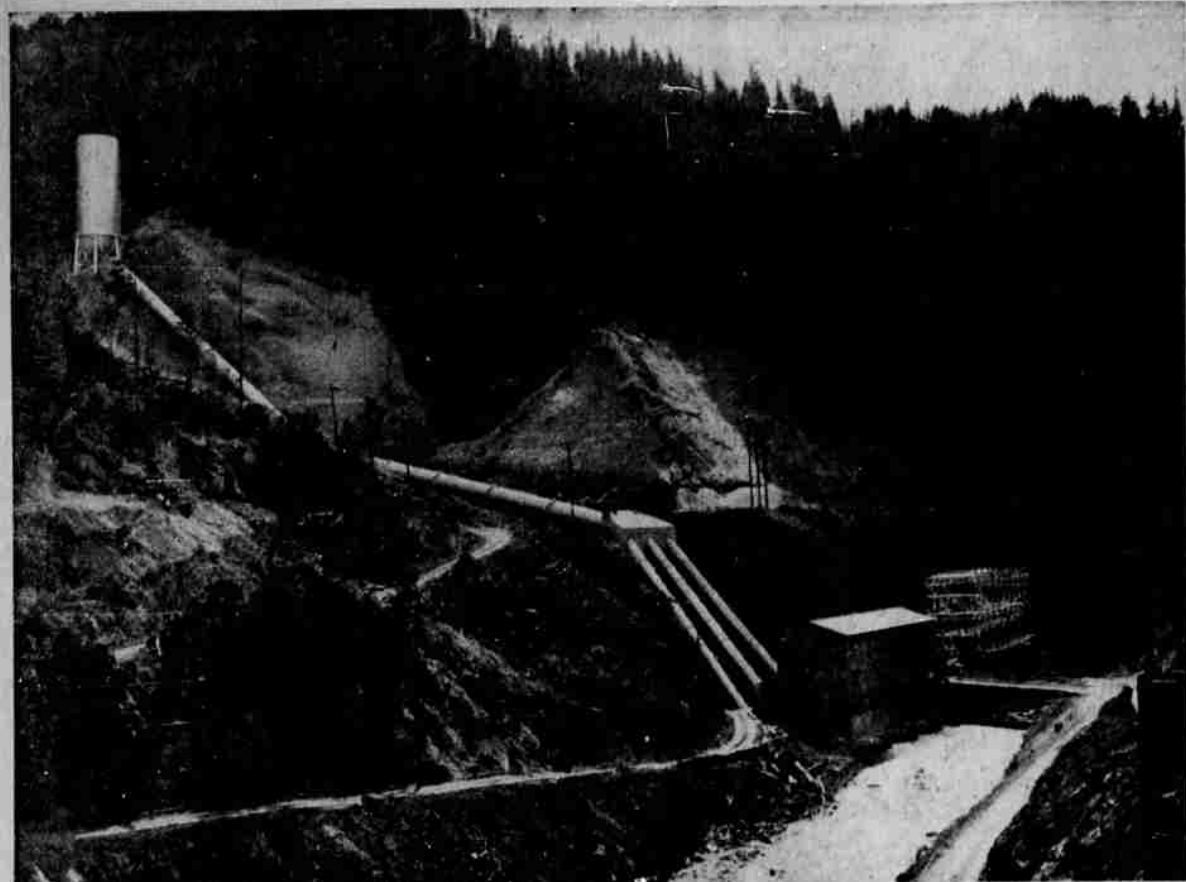
TOKETEE PLANT —Main unit of California-Oregon Power Company's power development on the North Umpqua River is the Toketee plant. This plant has a capability of 45,000 kilowatts and was the first to be built in the Umpqua power
