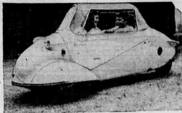
THEY FLIT IN A "FLITZER"—"Flitzer" is the name for this new German auto-scooter, being tried out by a couple of young women in Frankfurt, Germany. Fritz Fend, its inventor and manufacturer, is displaying it there. The tiny car, which can be entered only by swinging open the whole top, has been clocked at well over 60 miles per hour.
