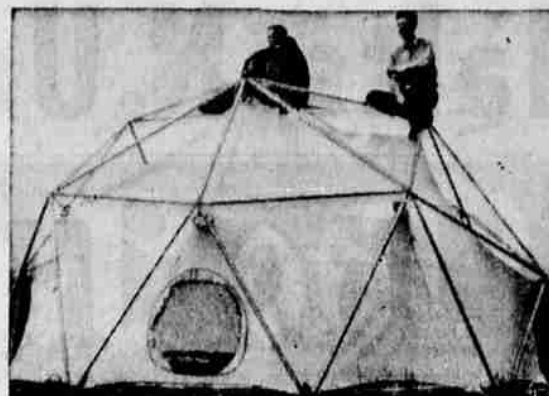
INSIDE-OUT TENT KEEPS STORMS OUTSIDE —This new-type tent, built inside-out so blizzards won't blow it away, will get a field test next summer when members of the Arctic Institute of North America visit the Pogy ice-cap on Baffin Island. Designed by Jeffrey Lindsay and Ted Pope of the Fuller Research Foundation, it consists of an aluminum tubing exterior framework from which is hung the tent. There are no interior support poles. The tent, demonstrated at Montreal, Canada, can be erected by two men in 25 minutes.
