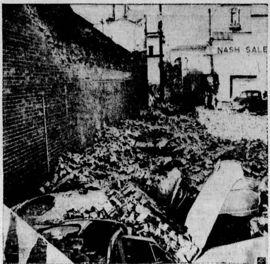
BUILDING TUMBLES — Thirty automobiles and trucks were covered when the building of a Fresno, Calif., garage collapsed. Fire department officials called to the scene attributed the destruction to heat expansion. The building had just been reroofed. No one was injured or killed, though only seconds before the crash, a man had parked a car next to the building. (AP WIREPHOTO)
