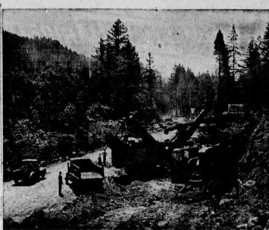
CONSTRUCTION crews are shown above hacking away at a big cut a mile south of Idelyd on a section of the new North Umpqua Highway. The project to pave and improve the road from Lone Rock Bridge to Rock Creek is scheduled to be completed by October. This view shows a section of the construction job looking west along the road. The $267,000 project is being built by the Funderburk Construction Co. of Sutherlin. (Picture by Paul Jenkins).
