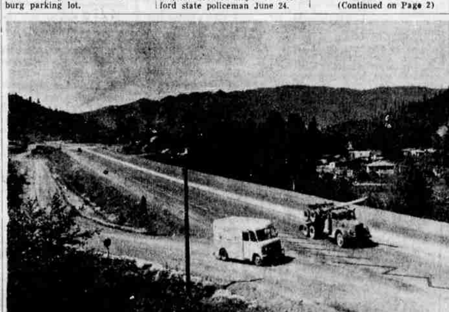
NEW CANYONVILLE bypass section of Highway 99 to direct through traffic around the town is shown above just after it was opened permanently several days ago. A $440,229 project of the Oregon State Highway Commission, this view looking north shows a truck at left coming onto highway after going through Days Creek underpass, one of two underpasses on the two-mile project, which includes a four-lane highway and broad traffic interchange facilities. Canyonville is at the right. Construction was started in November, 1950. Workmen began painting the traffic stripes today. (Picture by Paul Jenkins).
