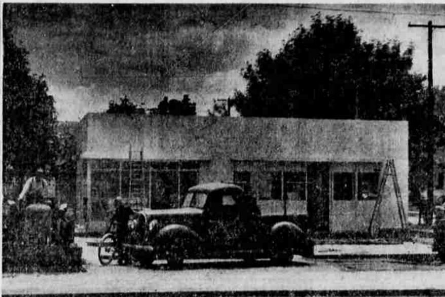
THIS MODERNISTIC new service station being built one block east of the Oak Street bridge will open shortly after July 1 with Verden "Bo" Boucock as station manager. A $30,000 project, it will have double islands with a total of four gasoline pumps. It will also have double lubrication bays. C. M. McDermott, Roseburg distributor for Tide Water Associated Oil Co., said ground will be broken this week on a duplicate station of the one above at a site on Garden Valley road across from Riverside School, where the Church of God was formerly located. (Picture by Paul Jenkins)
