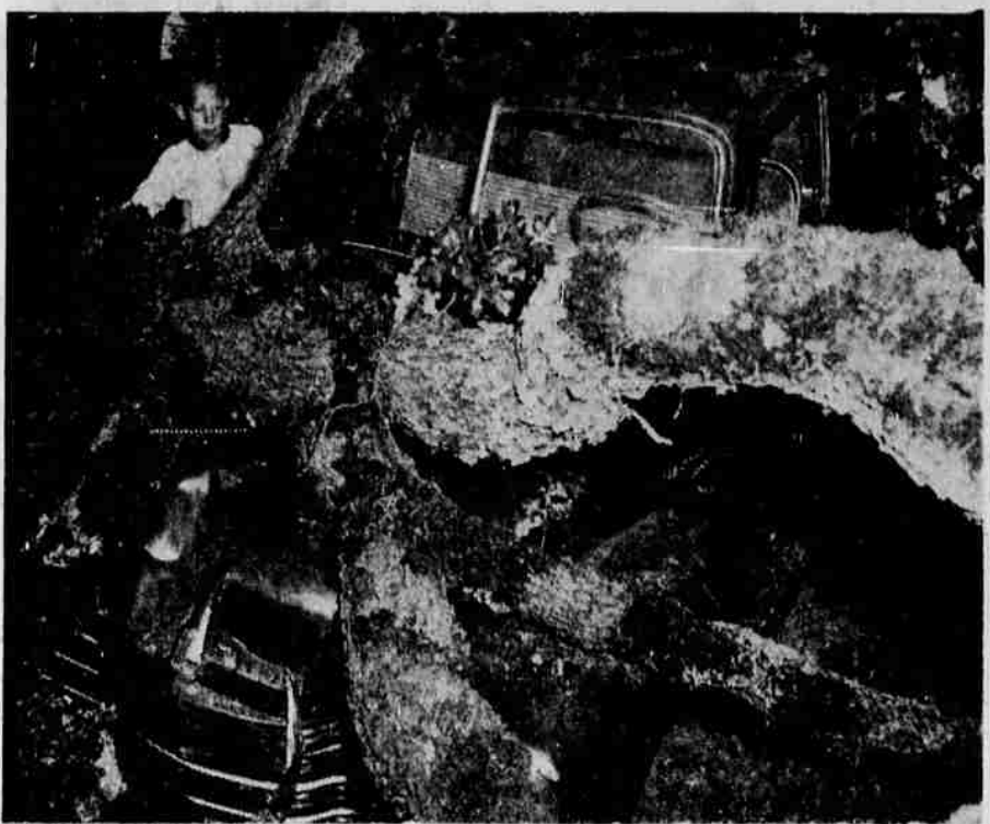
THE CLUTCHING HAND — Jim Barnhart, 11, inspects a crushed truck which two Roseburg women were about to enter late Friday seconds before the big oak tree crashed down into the yard of Mr. and Mrs. Gordon Marshall, 1314 W. First St. Rotted roots suddenly gave away and the huge tree tumbled into a yard where six children had been playing a half hour earlier. (Picture by Paul Jenkins)
