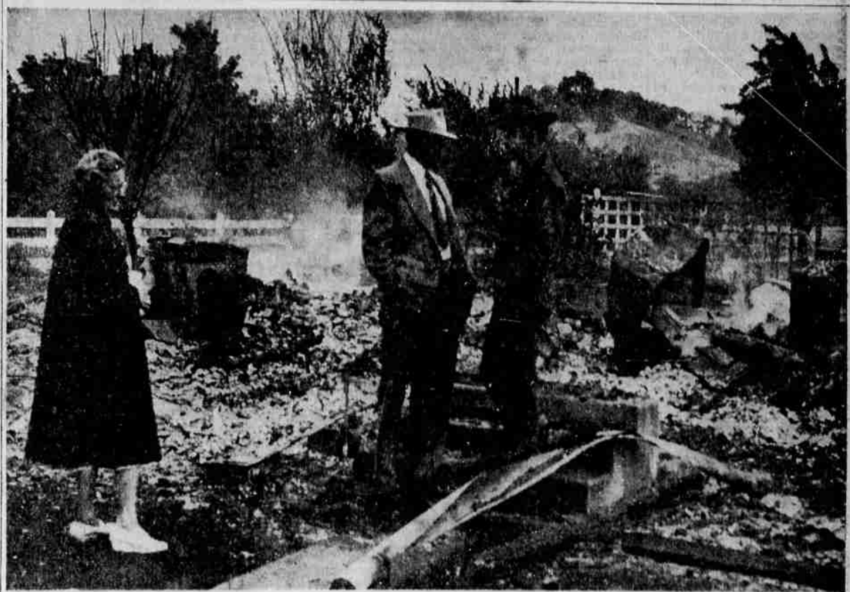
DEJECTED as they stand on the front door step of what was their ranch home near Wilbur, Mr. and Mrs. Harold D. McKay and son, Del, examine the smoldering ruins of the structure destroyed by fire Friday. Loss was estimated at
