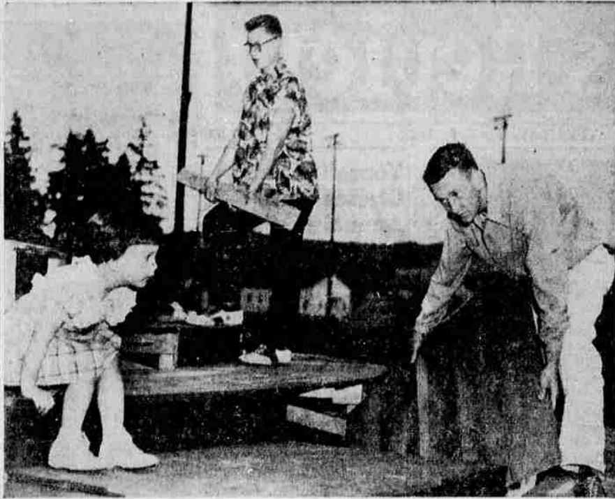
NEED SOME HELP? — Rita Martin, 3 1/2, gets ready to help Brian Booth, right, put finishing touches on the Queen's stand in preparation for the Senior High School May Fete, while Eddy Williams hauls a two-by-four into place. Both boys are working on the stand under supervision of Bill Sullivan. Fete was held at 8 p. m. Wednesday at the high school gym, under sponsorship of the physical education department. Paula Helweg is chairman. (Staff Picture)
