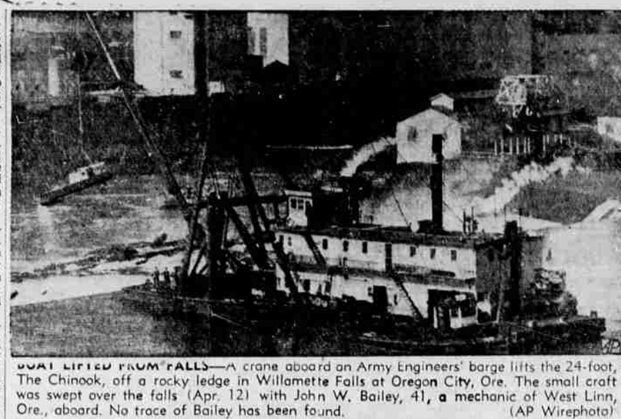
BOAT LIFTED FROM FALLS —A crane aboard an Army Engineers' barge lifts the 24-foot, The Chinoak, off a rocky ledge in Willamette Falls at Oregon City, Ore. The small craft was swept over the falls (Apr. 12) with John W. Bailey, 41, a mechanic of West Linn, Ore., aboard. No trace of Bailey has been found. (AP Wirephoto)
