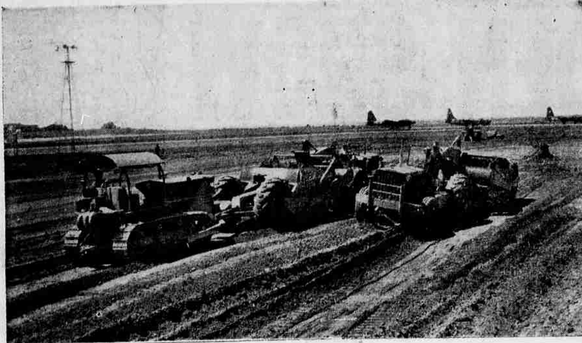
DRAMA IN DIRT: 23 yard loads boil into Peter Kiewit's new "Caterpillar" No. 20 scrapers and are hustled to the fill at 22 m.p.h. by "Cat" rubber-tired diesel tractors on Whidby Island naval air base runway extension. The DW 20's were supplied by Interstate Tractor and Equipment Co., local distributors, and are powered by new "Caterpillar" high-speed 275-h.p. diesels, have hydraulic-booster steering & air brakes.
