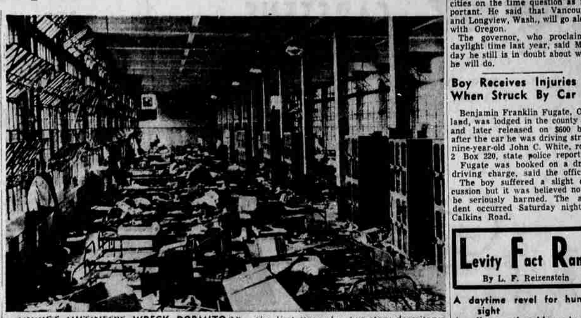
CONVICT MUTINEERS WRECK DORMITORY — The first floor of a two-story dormitory wing at the New Jersey State Prison at Rahway is shown littered with debris and wreckage while 231 convicts hold nine guards as hostages on the second floor, behind barricades. The prisoners evacuated the first floor (April 18), and centered their demonstrations on the second floor. Prison authorities permitted interior pictures for first time April 19. (AP Wirephoto)
