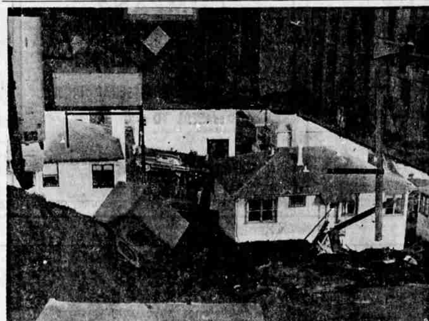
LOOK! NO BOTTOM —This is a basement-level view of the home of Mr. and Mrs. Robert Mayerson of South San Francisco, Calif. The sloping ground below slid away when Mayerson drove his car out to go to work and the floor of the garage disappeared down the hill. The automatic washer dangles in midair held by connecting rubber hoses. The hot water heater and wash basin are held by steel pipes over sheer space.
