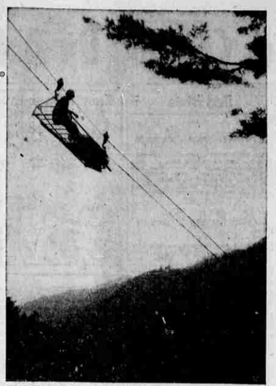
THE LINE IS BUSY—Riding high above the rugged mountain peaks on the Central Front in Korea, a U. S. soldier of the 7th Division uses an aerial tramway that hauls supplies to UN front-line troops. The high-wire transport system, rigged by U. S. engineers, hauls men and supplies with equal ease. (NEA-Acme photo by Staff Photographer Jim Healy.)
