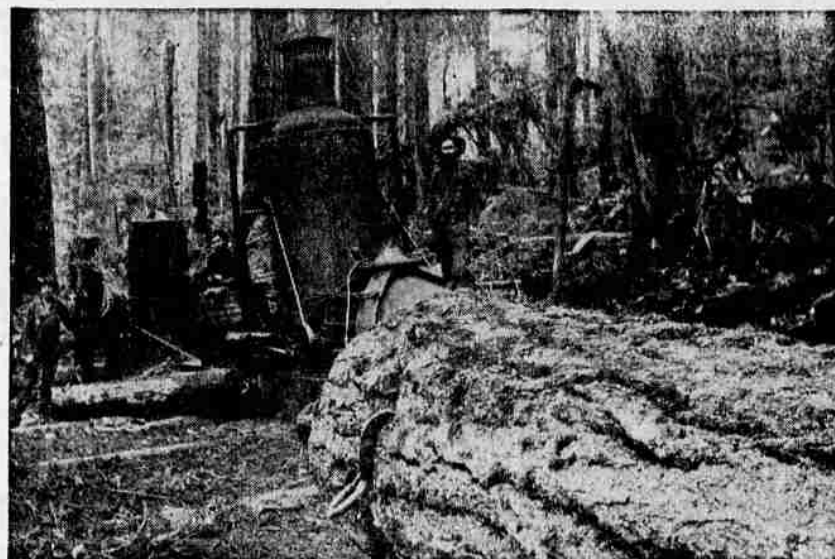
One of the first steam spool donkeys is shown in this authentic photograph (1898). The horse took up the slack and returned the line to the woods. It was about this time that the Skagit firm gained recognition as a repair and replacement shop for mills and camps, developed into a leading manufacturer of logging hoists.
