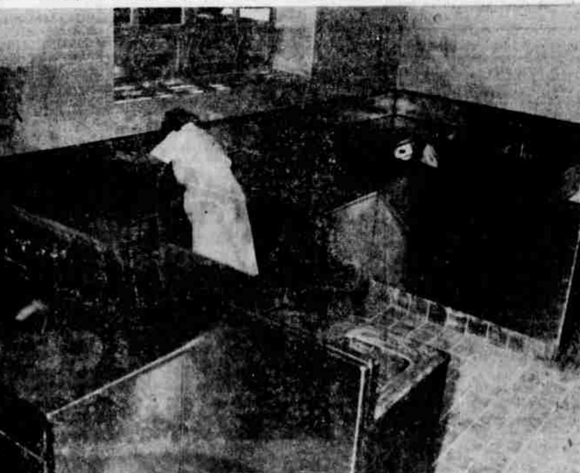
KITCHEN COMPARTMENTS for pastry, vegetables and meat are pictured as they are arranged in the basement of the new Mercy hospital addition. They are constructed of stainless steel. Kitchen has gas stoves and is arranged for direct line convenience. (Picture by Paul Jenkins)
