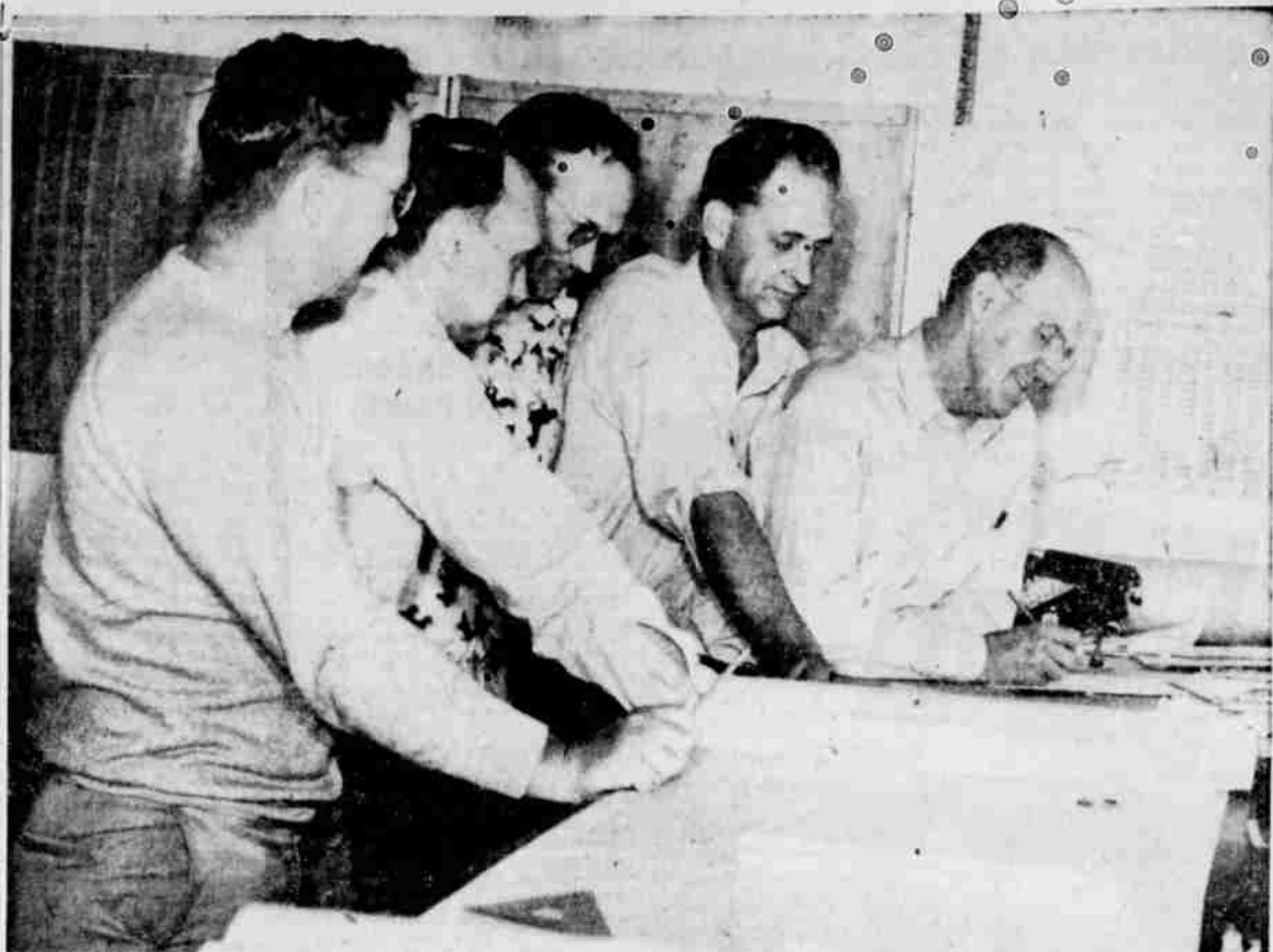
EARL PURDY, Jack Rowland, Roy Stein and Pat Gregory observe mission at its offices on Cobb street, engaged at the present time with interest as Larry Sullivan squiggles with figures over a drafting table. All are engineers employed by the state highway commission in preparing estimates for various construction jobs. (Paul Jenkins)
