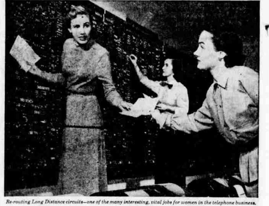
Re-routing Long Distance circuits—one of the many interesting, vital jobs for women in the telephone business.
