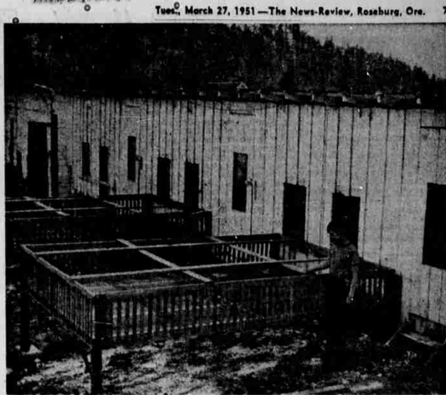
BROODER RUNS —Jim Conn, young son of Jay Conn, stands beside a brooder run, one of many such forming a part of the extensive brooding facilities in the Conn Hatchery at Melrose. The runs have wire-mesh floors and sanitation necessities. —(Paul Jenkins)
