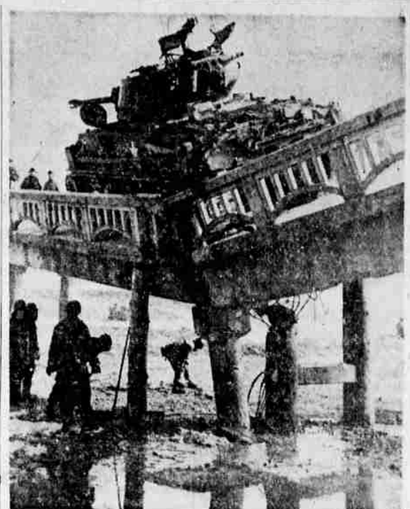
PUSH HIM UP, JOE —These engineers of a 1st Cavalry Division battalion must have a lot of faith in their work as they stand under weakened bridge near Yangzi, Korea, to shore it with logs. The M-4 tank that caused the structure to sag will sit there until a tank retriever arrives to remove it. (NEA Telephoto)
