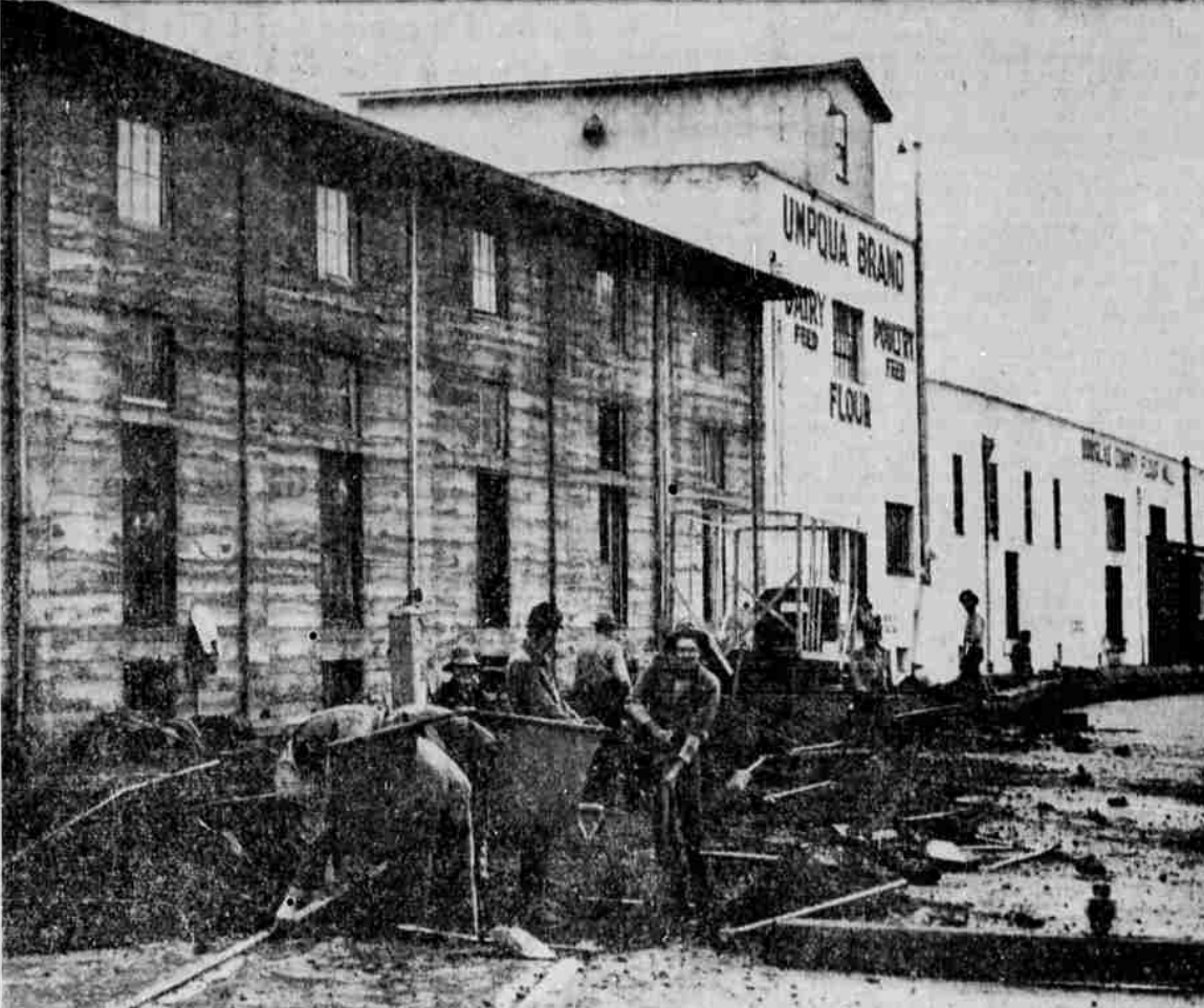
A SOUTHERN PACIFIC section crew tears up track on a Sheridan street siding between Oak and Cass streets serving the Douglas County Flour Mills, preparatory to laying a new bed for the rails. "Railroad people here speak of this as the 'Abe' spur," recalls C. P. Moody, S. P. agent. "I don't know why. Named for some of our old-timers, probably."
