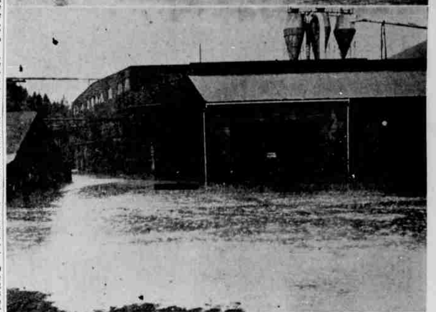
FLOOD SCENES FROM MYRTLE CREEK —Top picture shows Highway 99 just south of Myrtle Creek. Center picture shows a view of the Weaver addition just across the bridge south of Myrtle Creek. The houses were under three to four feet of water. Bottom picture shows the Firmco Plywood mill at Myrtle Creek during the height of the flood. (Picture by Ada's Photo Studio, Myrtle Creek.)
