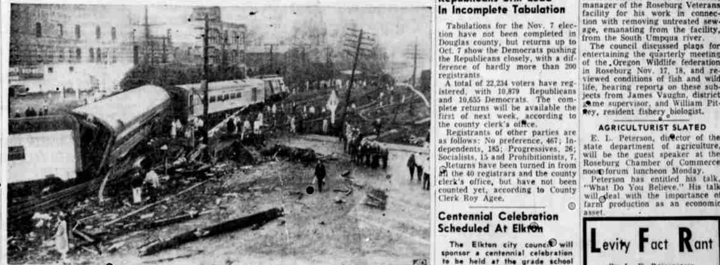
WHERE TWO TRAINMEN DIED —This is a general view of the wreck of the New York Central railroad express "North Star". The engine and 11 cars were derailed in the heart of Oneida, N.Y., when the train hit a steel freight door which had fallen across the tracks. Note the twisted steel rail in right background. Two trainmen were killed and several passengers injured. (AP Wirephoto.)
