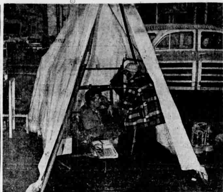
CABLE SPlicERS —Working under a telephone company tent shelter are cable splicers Thomas McGill, left, and Arland Thornell. Their job is the intricate work of splicing the myriad of wires making up a telephone cable. The work is part of the Pacific Telephone and Telegraph company's program to convert the city of Roseburg from manual to dial telephones. This is expected to be completed early in 1951. (Picture by Paul Jenkins.)
