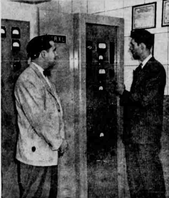
RADIO ENGINEERS Ralph Smith and Leo Reetz, left, stand before the transmitter in the control room of Roseburg's new radio station, KRXL, which went into operation on a "check up" basis Tuesday evening. Reetz, tabbed at KRXL as announcer-engineer, comes to Roseburg from KRUL, Corvallis; KNPT, and KASH, Eugene. In addition to radio station experience, he also owned his own radio service shop in Corvallis. (Paul Jenkins photo.)
