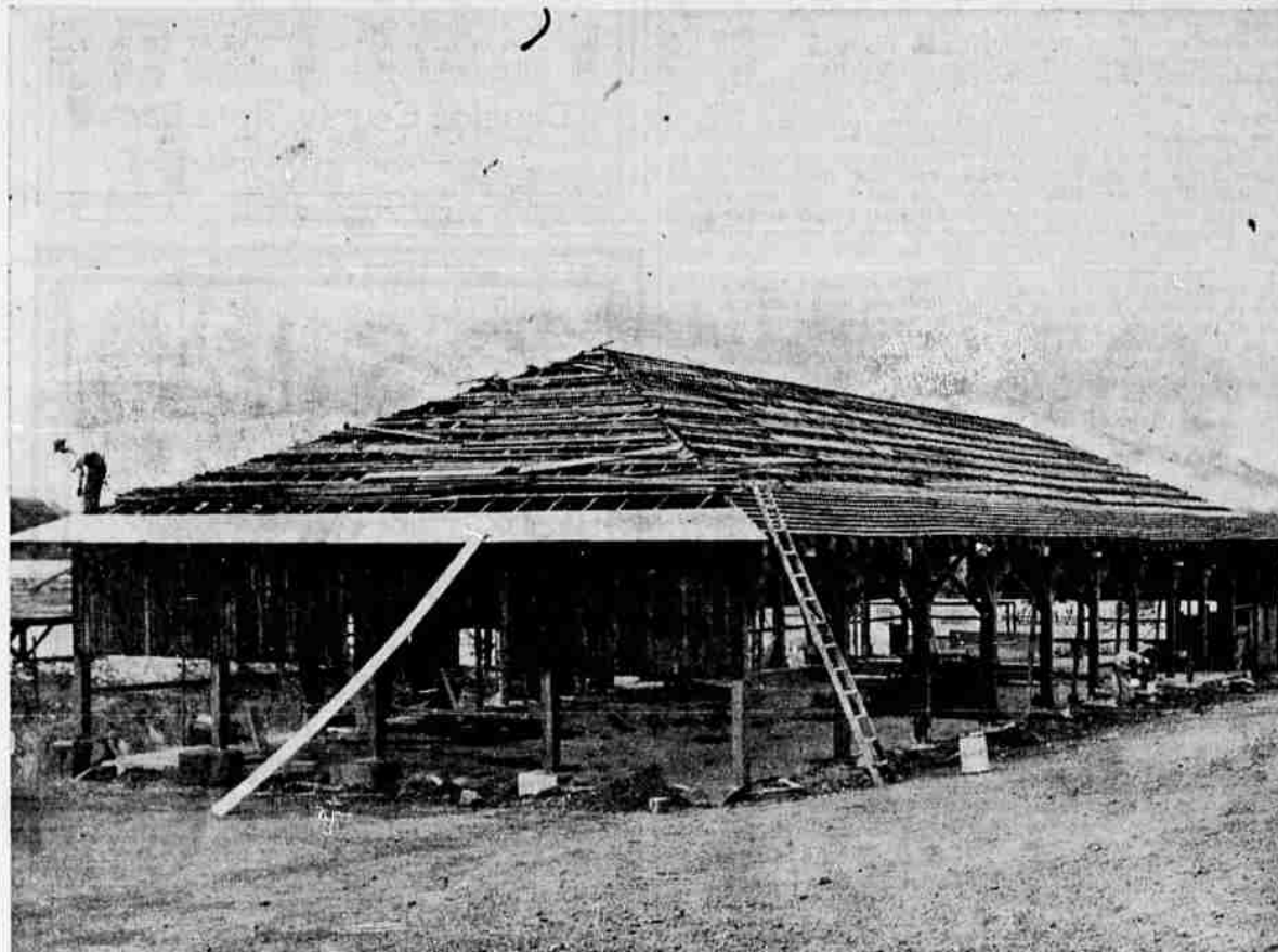
BENSON grade school playedshed was to receive a new shingled building was erected almost 30 years ago. To keep a new roof this summer in preparation for rainy school days ahead, from collapsing, workers must also repair the foundation, replacing many of the posts. When workmen inspected the structure closely, they found termites had almost undermined the foundation posts since the
