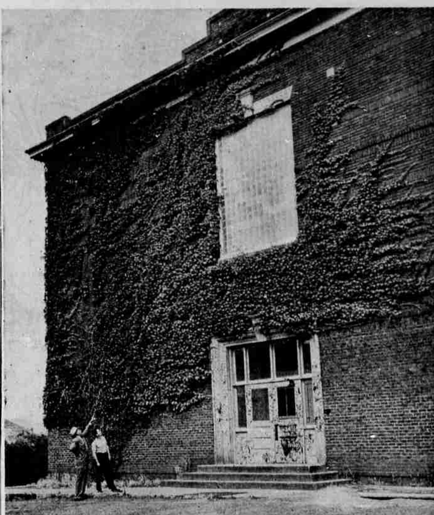
BENSON school also came in for some revamping when workers installed this large glass block window, replacing one of regular design. Supt. Elliott and Principal Roy Crain point out the remodeling, installed on the "noisy" end of the building. The city school board hopes the glass block will make teaching easier, with noise from nearby sawmill eliminated.
