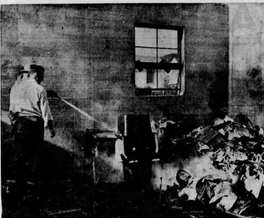
FIXTURES FIXED —City firemen spray water on plumbing fixtures, bowls, basins and other plumbing supplies scheduled for installation in the new county home before fire destroyed much of the material Thursday afternoon. Fire Chief William Mills blamed a careless smoker for providing the spark to set boxes and packing ablaze. (Staff photo)
