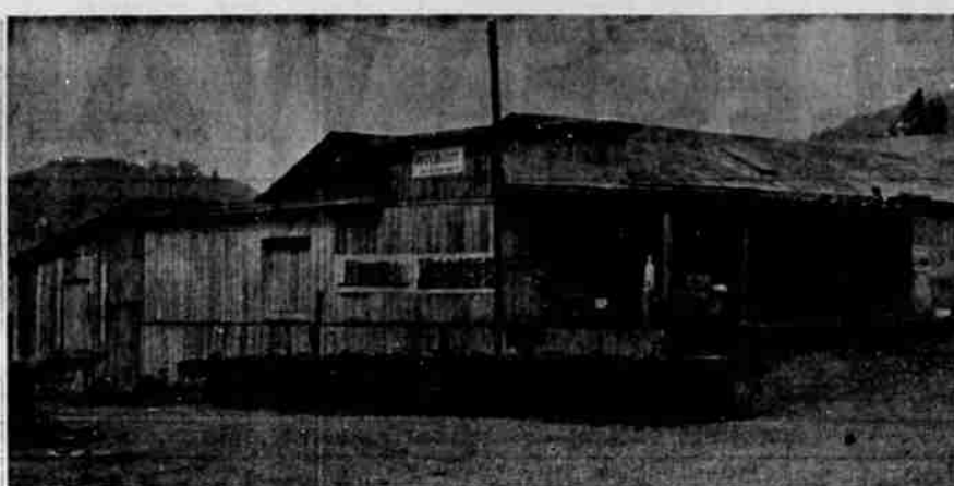
BEFORE FIRE broke out in the old warehouse of the Flegel Transfer and Storage company, the building looked like this. Used principally for storage, the structure also housed mechanics tools, a truck and various other items, all of which were lost. (See also story and picture on page one. Paul Jenkins photo)
